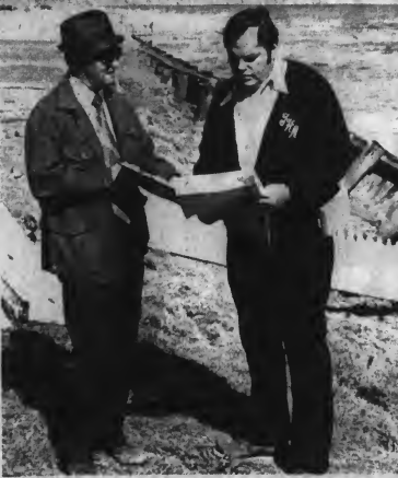
John Graff (left) and Tom Nichols discuss inspection of storm damaged bulkhead to determine City's qualification for disaster relief aid.
